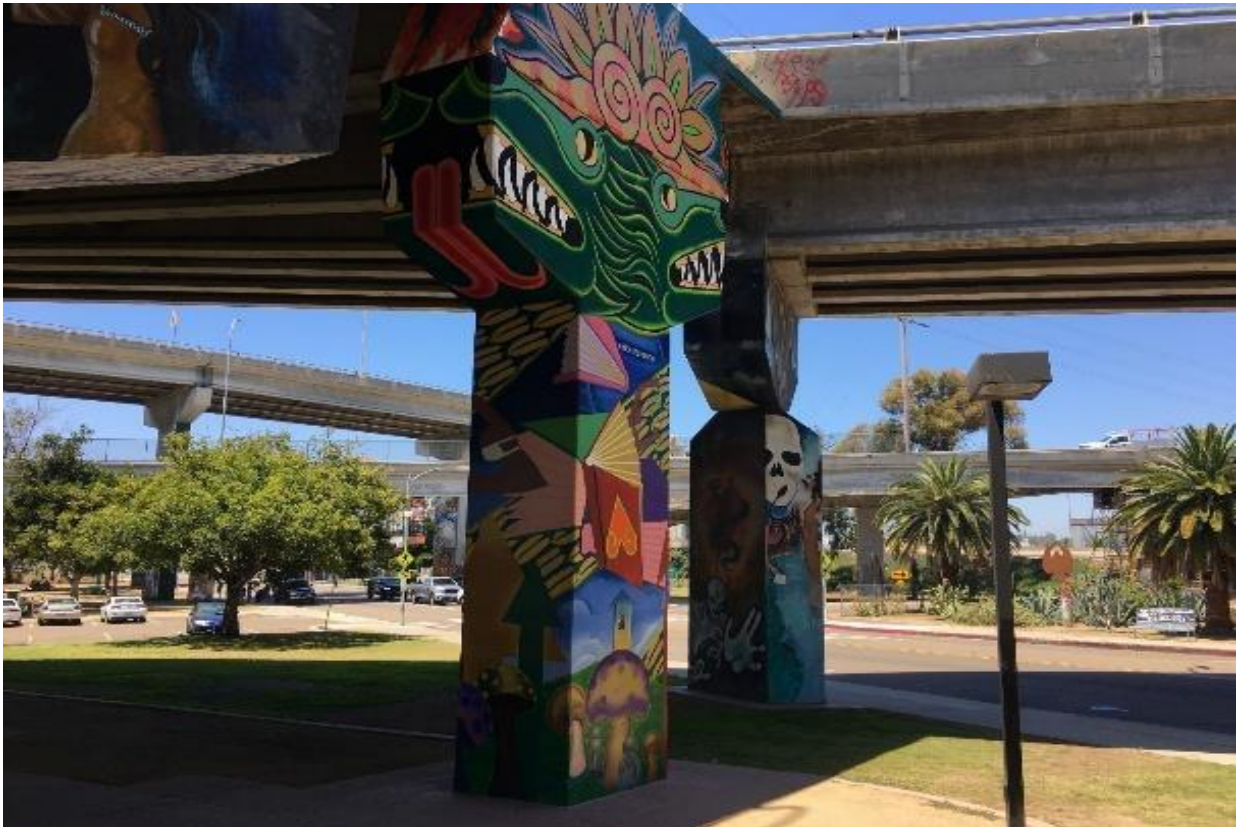
Figure 1: The bridge pillars of the Coronado Bay Bridge and the Interstate I-5 in today's Chicano Park in San Diego: on the one hand a symbol of spatial appropriation of the Mexican-American community, on the other hand a sharp divide and borderline between downtown and the neighborhoods of Southeast San Diego, which are characterized by a lack of symbolic capital. Source: Albert Roßmeier 2019
